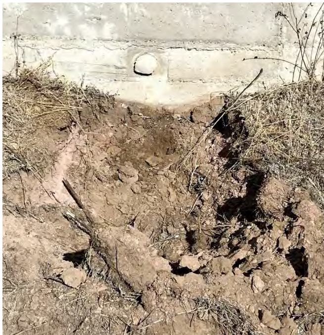
Photograph No. 4 Excavation Beneath a plugged drain pipe
