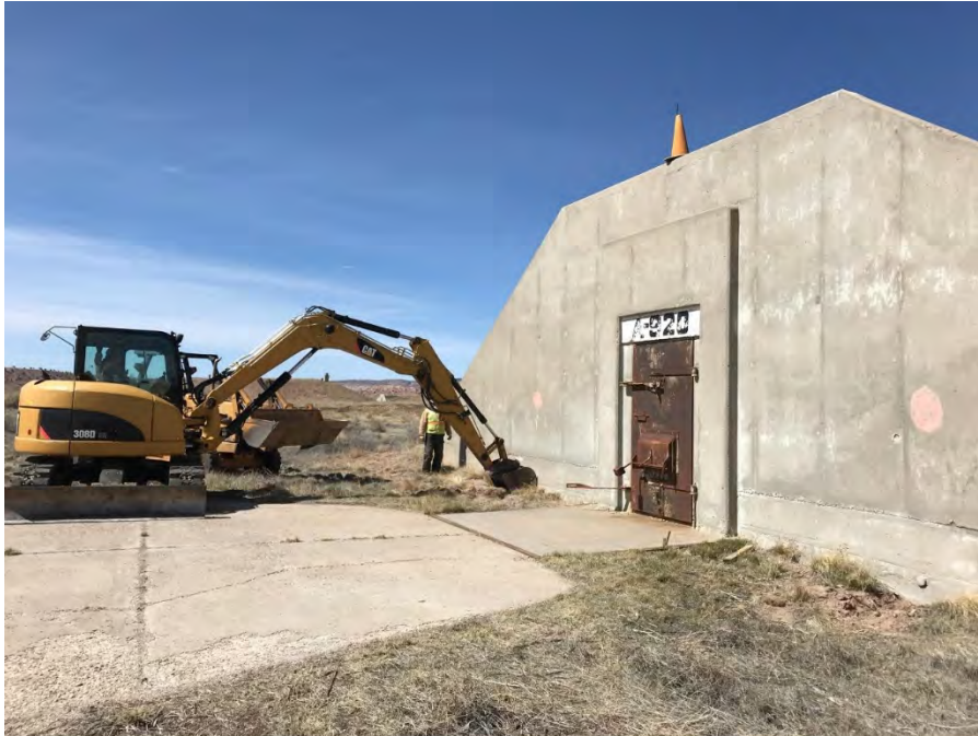
Photograph No. 3 Excavation at Igloo A-920
